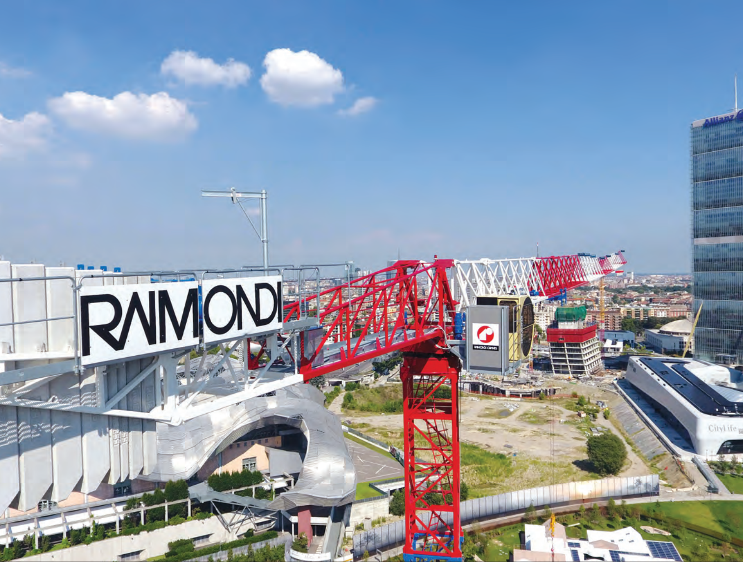
The Raimondi MRT234 topless tower crane erected in Milan, Italy
